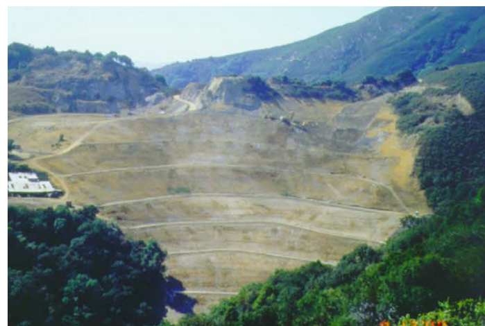
Top: Before remediation of Gambonini Bottom: after remediation of Gambonini
