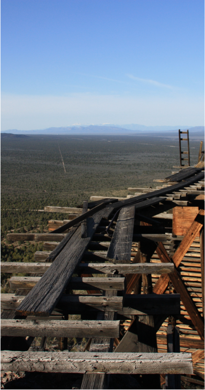
Ore Loadout, Lincoln County Nevada
