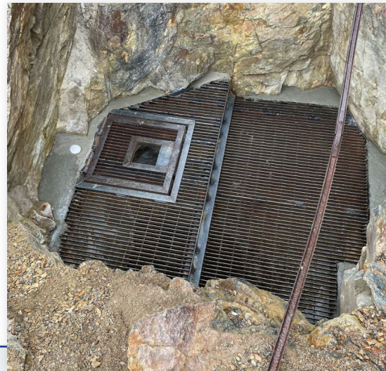
Below: Sealed mine shaft in Boulder County, CO.
