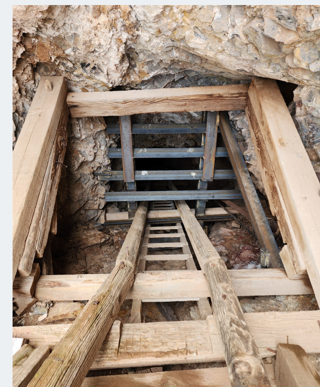
Before and after safeguarding steep mine entry in Death Valley National Park, Inyo County, California
