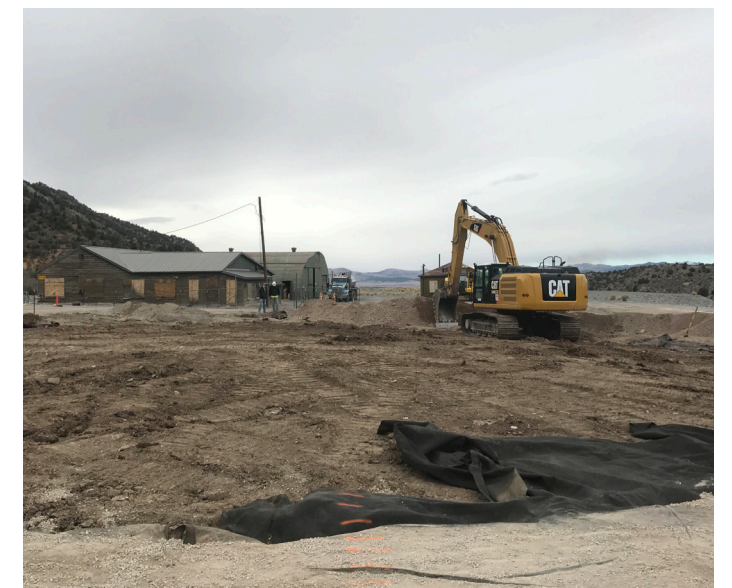
Backfill is complete. Preparing to replace the cap of geotextile and crushed limestone.
