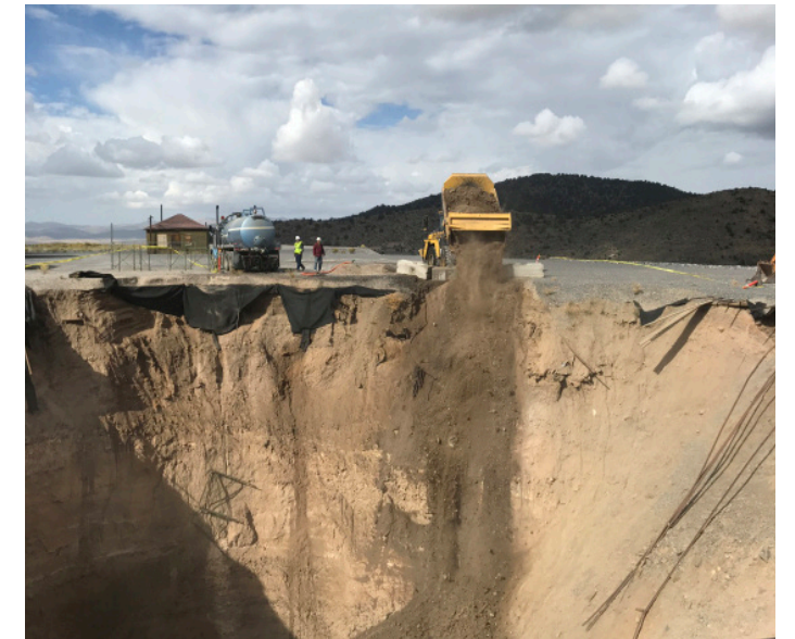
Early stage of the dumping of repository waste to fill the subsidence.
