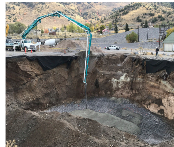
Construction of reinforced concrete plug on top of leveled fill. Once the concrete cured, additional fill material was placed and compacted to near the surface.
