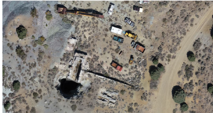
Over head image of Forman Shaft before closure. Note the size of the shaft compared to the abandoned equipment on the site.
