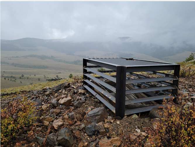
Bat Cupola closure over mine shaft, Carbon County, Wyoming
