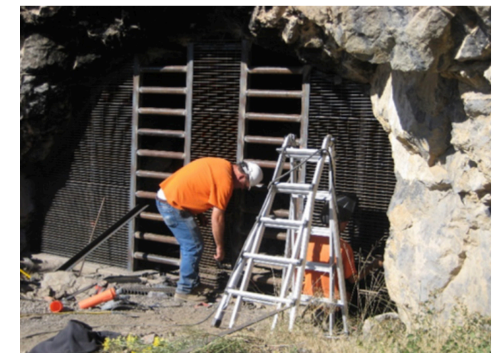
Bat Accessible Closure, Fremont County, CO.
