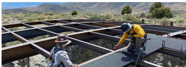
Installation of expanded metal grating over the cupola structure
