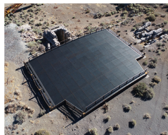
Completed cupola over Forman Shaft
