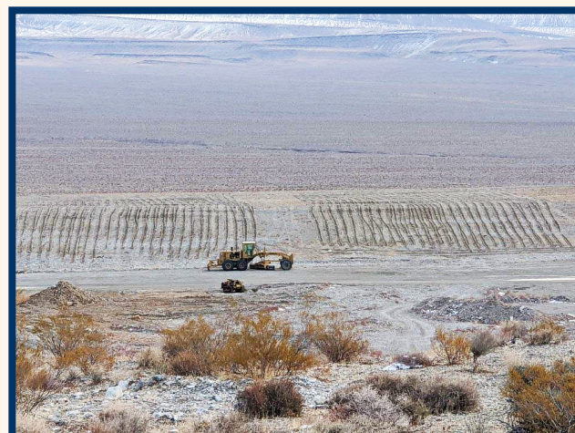
Test plot construction at the Sterling site near Beatty. Coeur constructed two one-acre plots using media from the Wood Canyon Fm.
