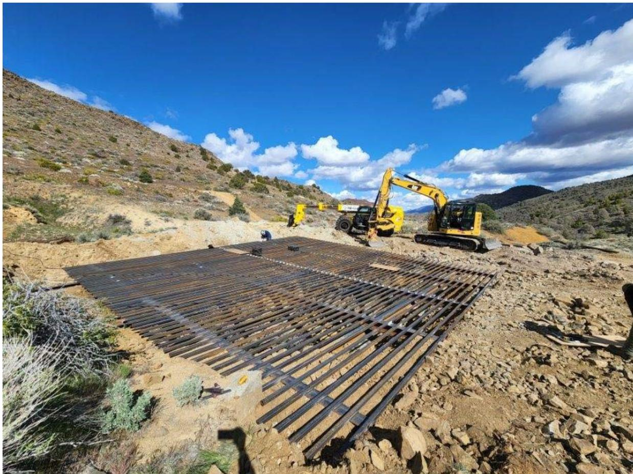
Photo 5 – EPS installing wildlife compatible and culturally sensitive grate at Sutro Airshaft #4, during the VC Grand Prix hard closure project.
