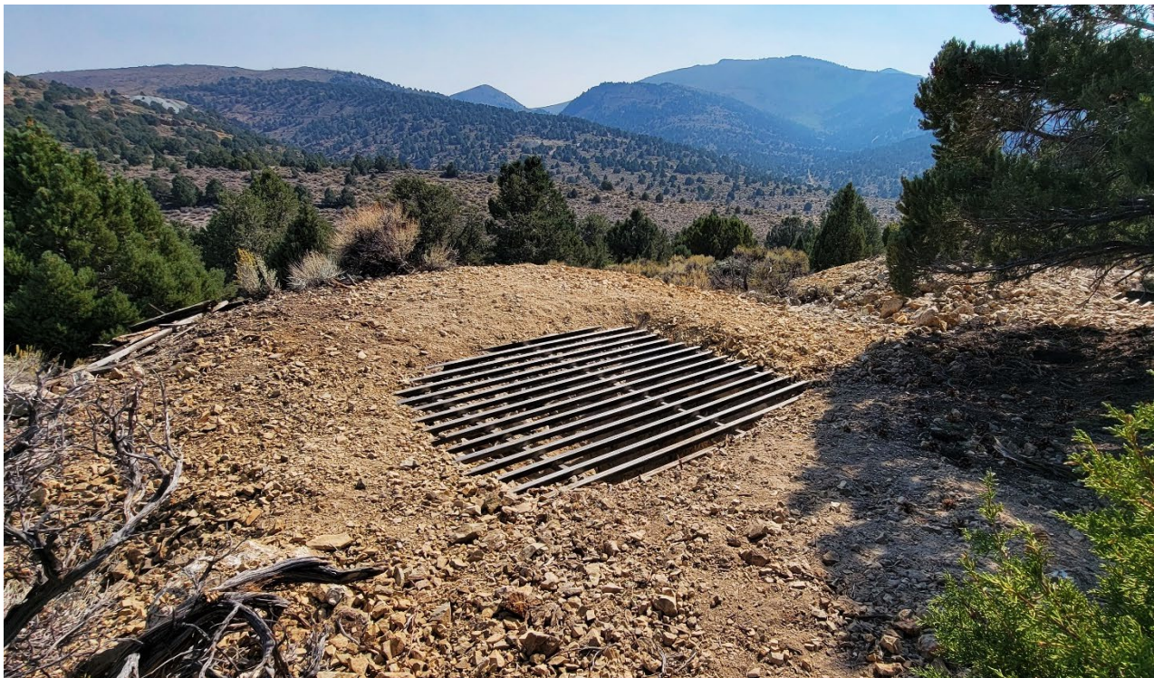
Photo 9 – AML closure by EPS for US Forest Service in Mineral County.
