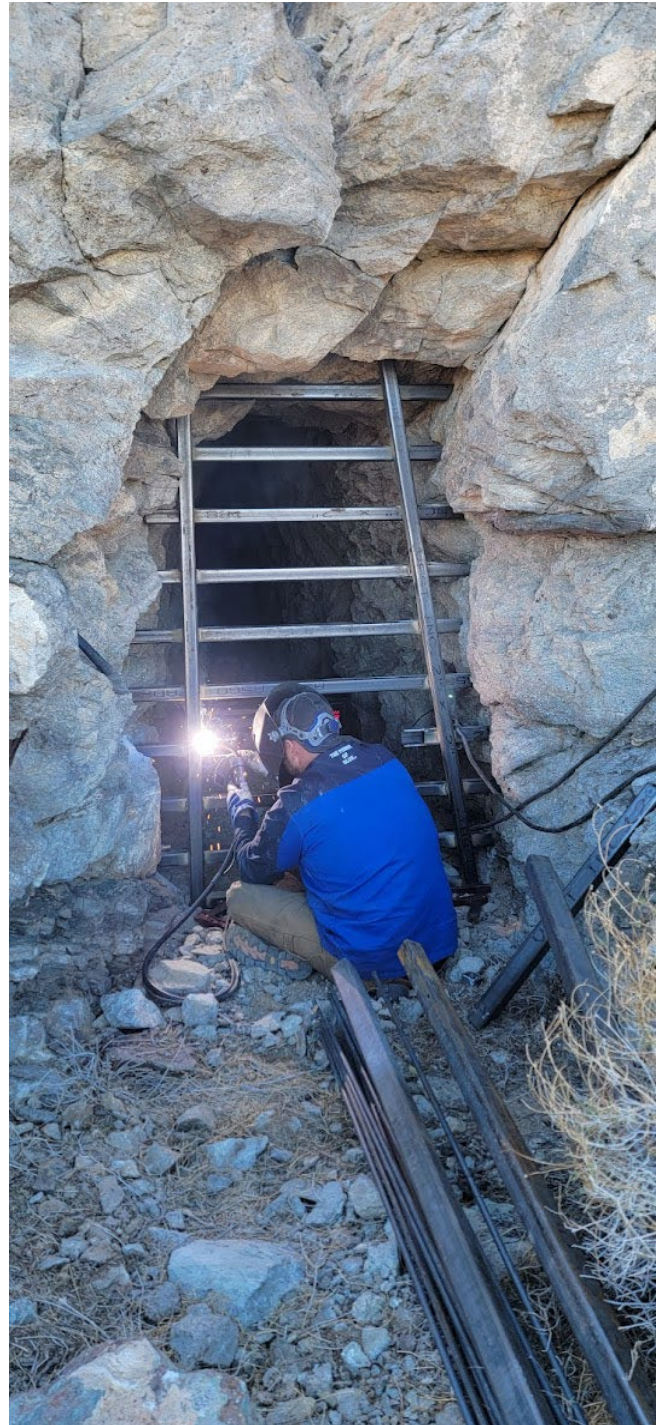
Photo 6 – EPS staff welding steel bars on a wildlife-compatible permanent closure at Copper Butte, Clark County.
