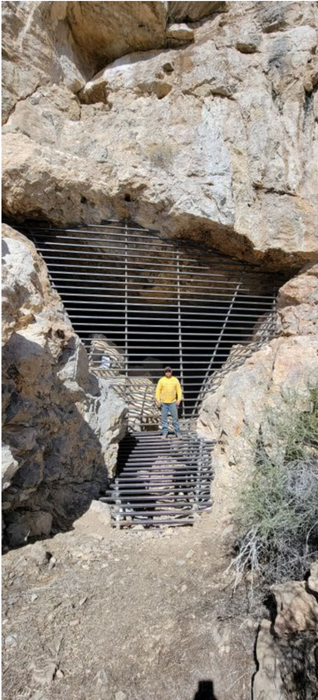
Photo 7 – Wildlife-compatible closure at historic Potosi Mine Site, Clark County.
