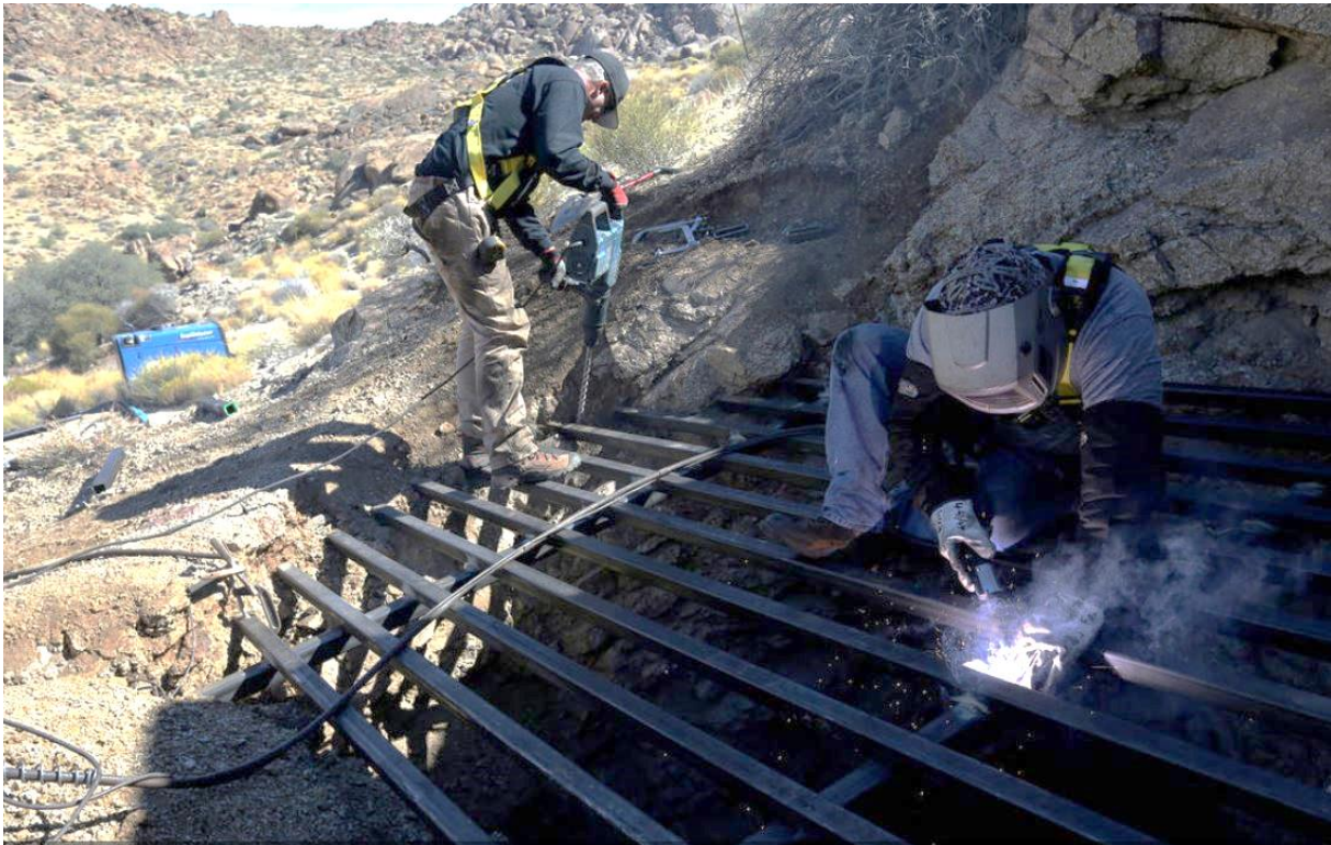
State Contractor, Environmental Protection Services, constructing a wildlife compatible closure in Gold Butte National Monument, Clark County
