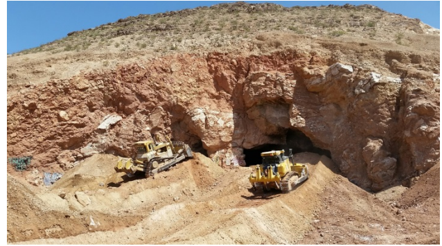
Two D-10 dozers backfilling adits at the Arden Closure project, Clark County
