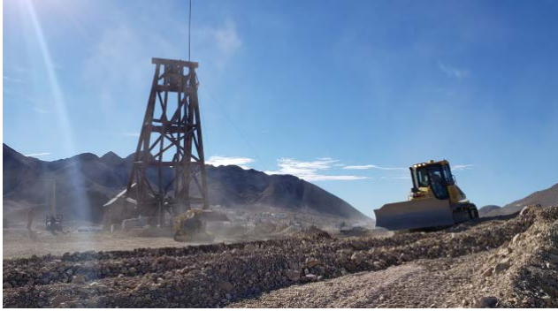
The Division Contractor, EPS, re-contouring the Silver Top waste rock dump for the future headframe restoration, Nye
