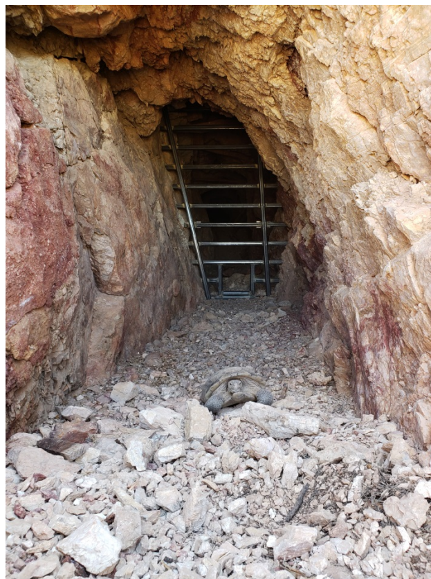
A desert tortoise exiting the recently installed bat gate with a tortoise door at the Gold Butte closure project, Clark County, October 2018
