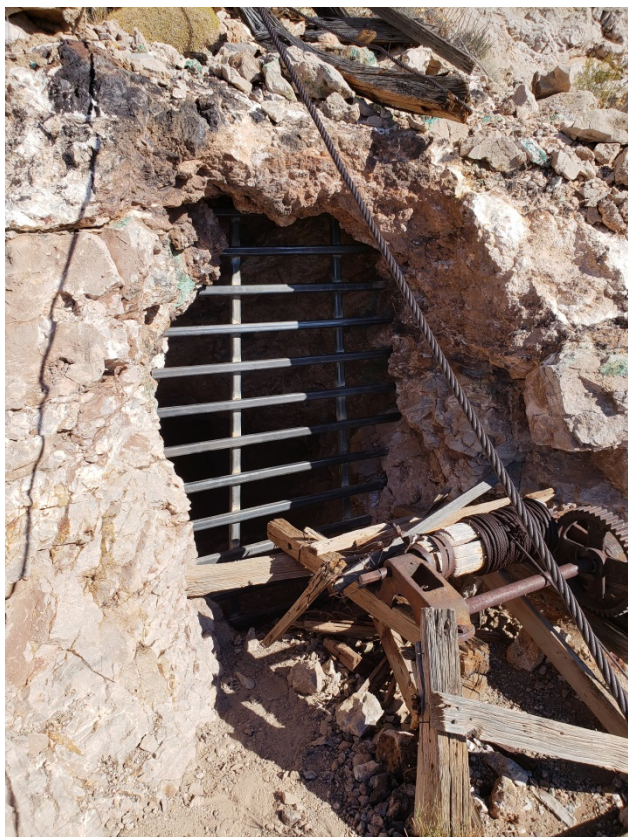
Bat gate installed at the Gold Butte closure project, Clark County, October 2019
