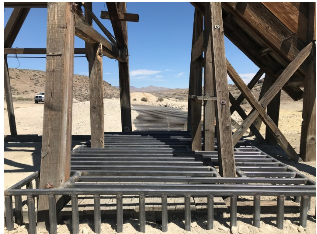
Bat Compatible cupola over the main shaft at the Broken Hills closure project, Mineral County
