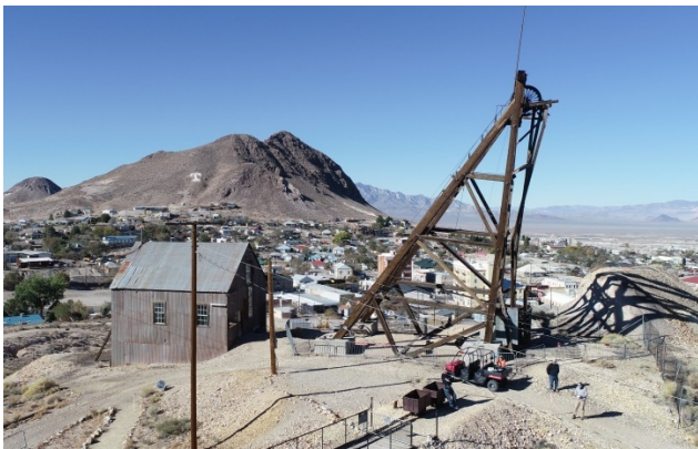
Before photo of the Silver Top headframe showing the lean, in October 2018, Nye County.
