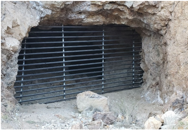
A 22' wide by 13' tall bate gate at the Gunmetal Complex, Mineral County.
