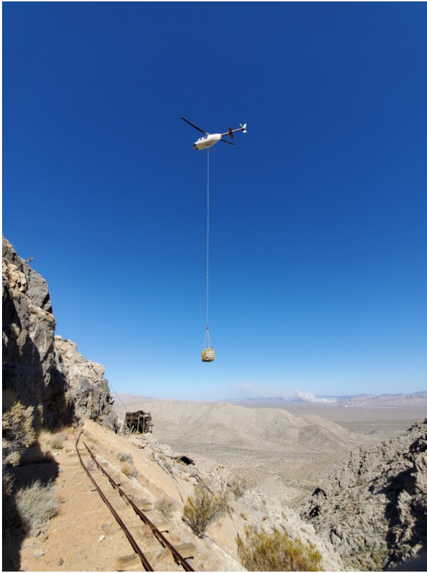
Helicopter slinging a load of materials to the portal of one of the Goodsprings project adits. In the foreground are the ore cart rails leading to the ore bin and remnants of an aerial tramway that once led to the bottom of the hill, Clark County.
