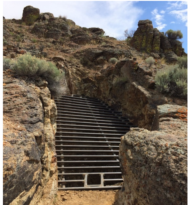
Bat grate with owl access for roosting, Washoe County.
