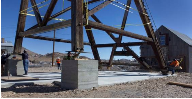
The Park's Contractor, Simerson, placing the reconstructed Silver Top headframe into place on the new foundation, Nye County.
