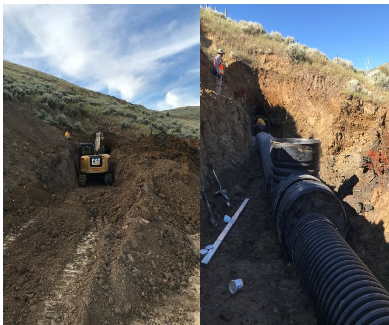
Left photo: EPS excavating the Birthday Mine. Right photo: The culverts being installed, Humboldt County.
