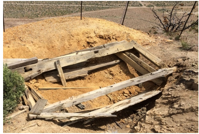
After photo of a completed polyurethane foam closure with the collar timbers still intact, Washoe County.
