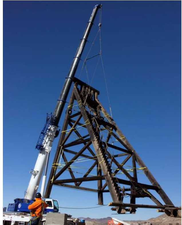
The Park's Contractor, Simerson, lifting the reconstructed Silver Top headframe to place on the new foundation, Nye County.
