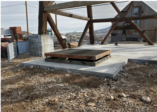
The bat cupola built by the Division's contractor, EPS, covering the 1,200' deep shaft, Nye County.
