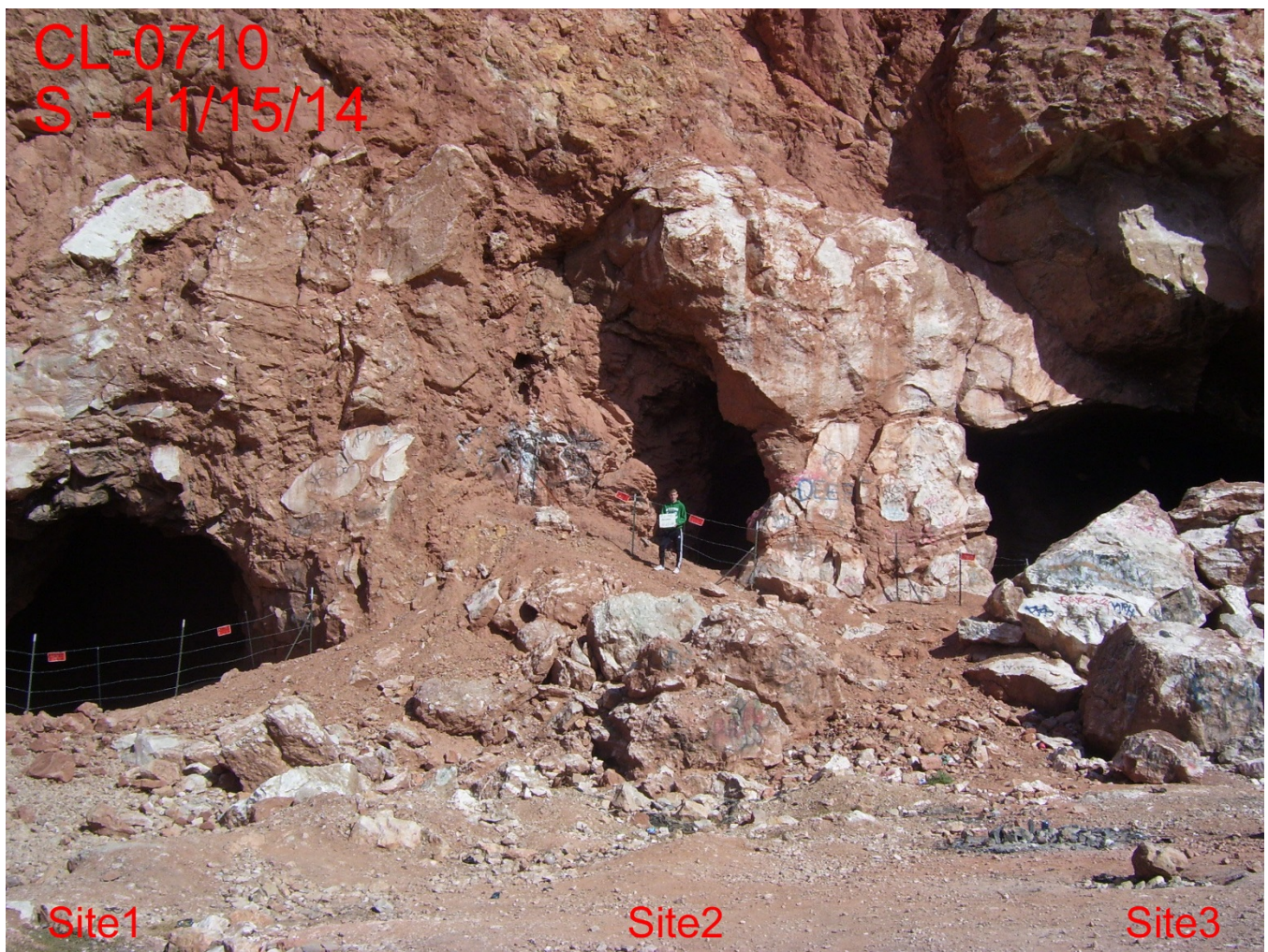
Image 2. Photograph of several abandoned mine hazard openings at the Arden Mine site. This photo was taken during an Eagle Scout project in late 2014, and has been vandalized and repaired multiple times since. Temporary barriers have been deemed ineffective, and a more permanent solution is being discussed with the Clark County Real Property management group.
