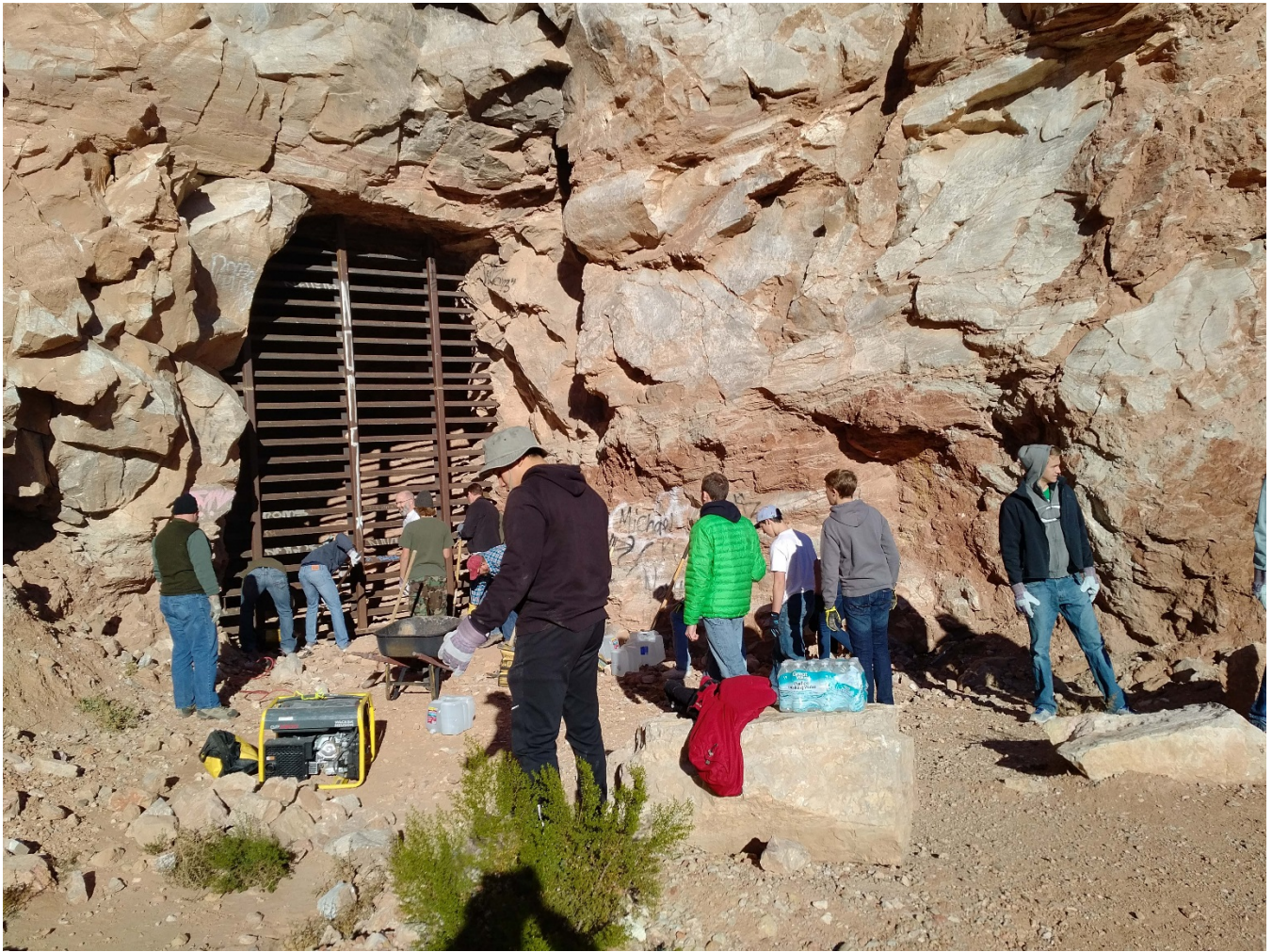
Image 3. Eagle Scout project from December, 2016. A bat gate at the Arden Mine was compromised by a large hole dug beneath the gate. For this Scout's project, a concrete footing was dug and poured beneath the gate, reestablishing integrity of the securing.
